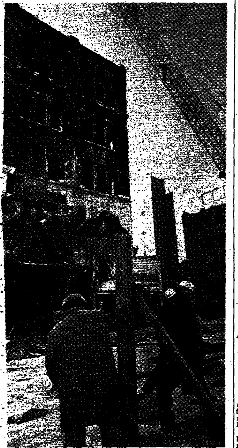
The gutted store at 520 Fulton Street in Brooklyn, workmen build that will be placed around the building before it is demolished.
